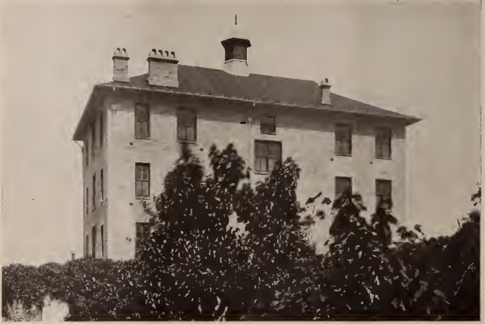
New Woman's Ward of Kashing Hospital, Built in 1917. Known as the B. M. Palmer Memorial Hospital.
